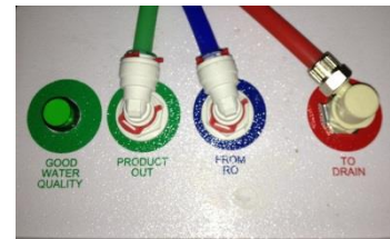
Top view of Divert-to-Drain showing tube connections
