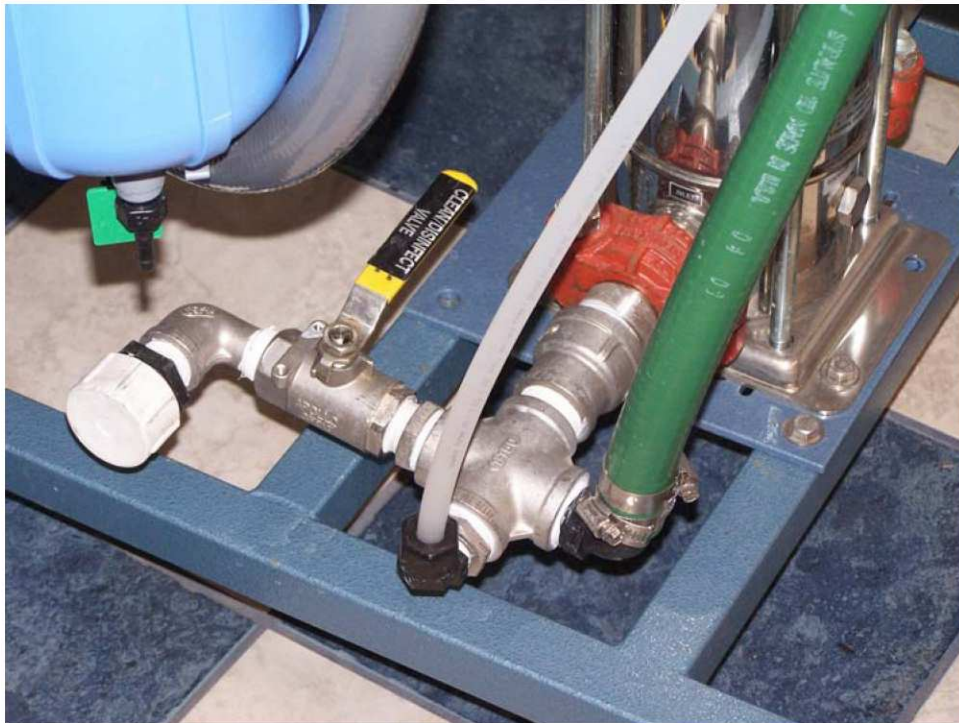
Diagram ROIPA 1 Pump Inlet Header located on left side of RO at the bottom.
