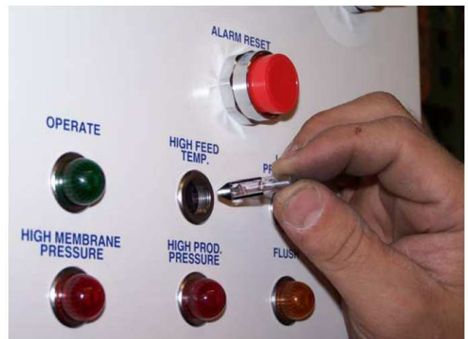
Diagram BLC2 Showing Bulb Removal / Installation
