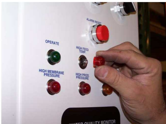
Diagram BLC1 Showing Lens Cover Removal / Installation
